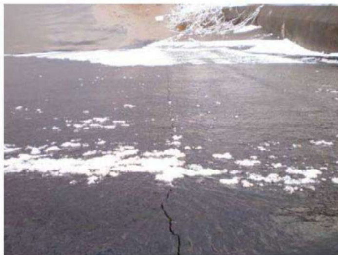
Figure 7 Asphaltic concrete face of Minamikawa Saddle Dam
