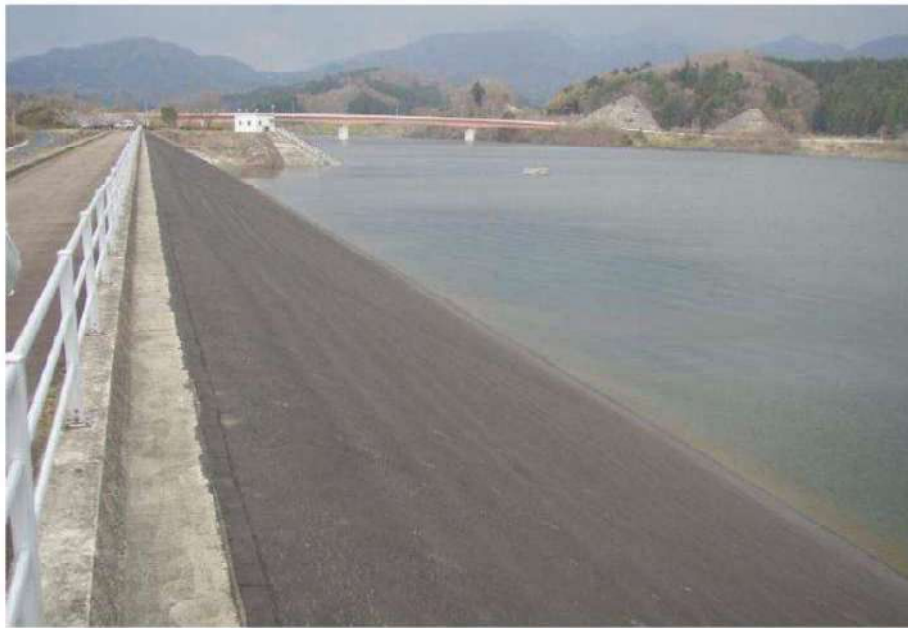
Saddle dam: asphalt concrete face rockfill
