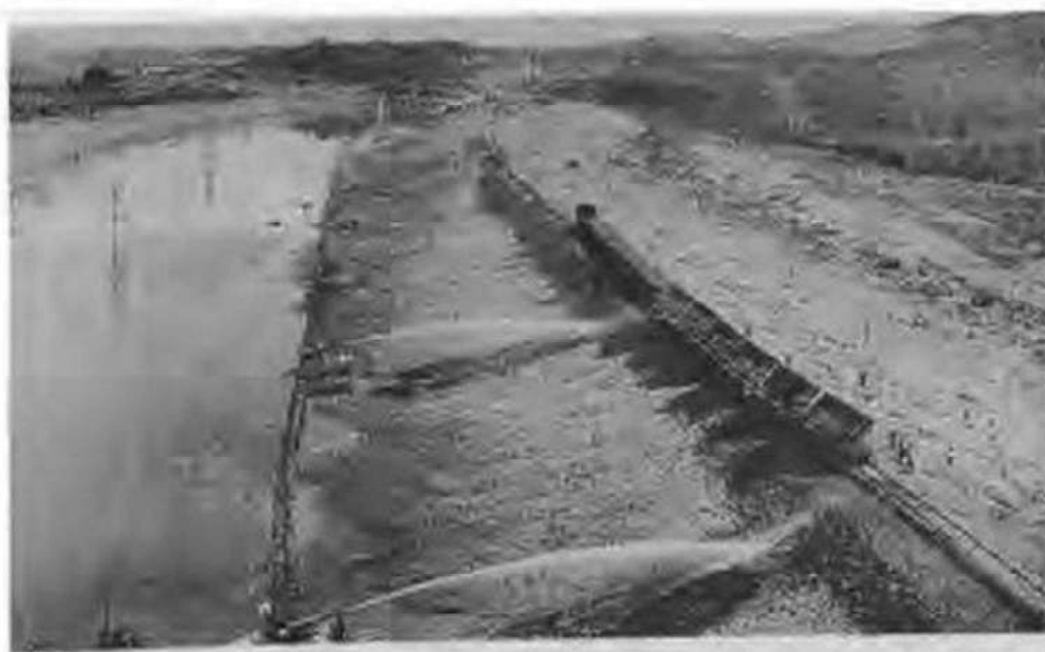
Photo 1 Embankment Construction: Material dumping and Water Jet Washing
